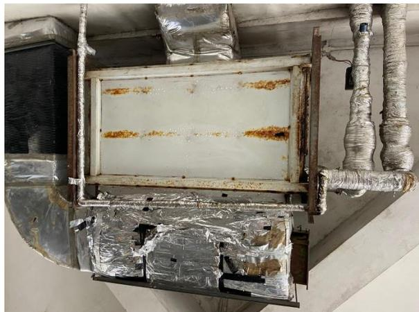
*Gambar 3. 13 Fan Coil Unit*
