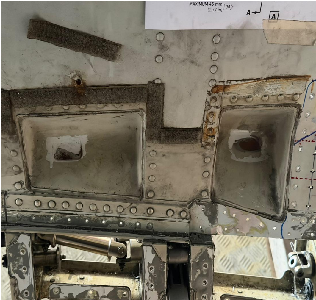
Lampiran B Defect Inner Skin Aft Cargo Door
