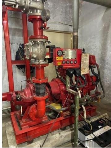
Gambar 3. 24 Diesel Engine Pump
